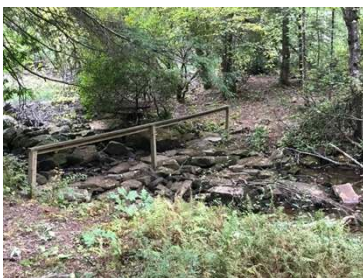
A stone bridge with wooden rail
